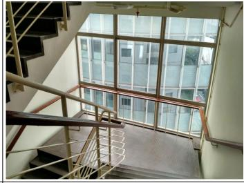
(g) The original fire escape staircase with old fittings and setting, terrazzo dado finishes and timber railings at the end of the short block 位於短翼末端原有的走火樓梯,包括其舊式配件及環境、水磨石牆裙及木欄桿
